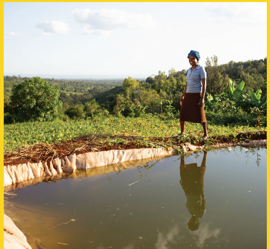
100m 3 rainwater harvesting pan that holds around 100,000 litres of water.
